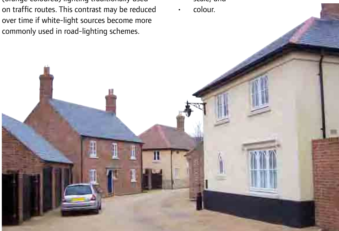
Figure 10.3 Street light mounted on a building.
