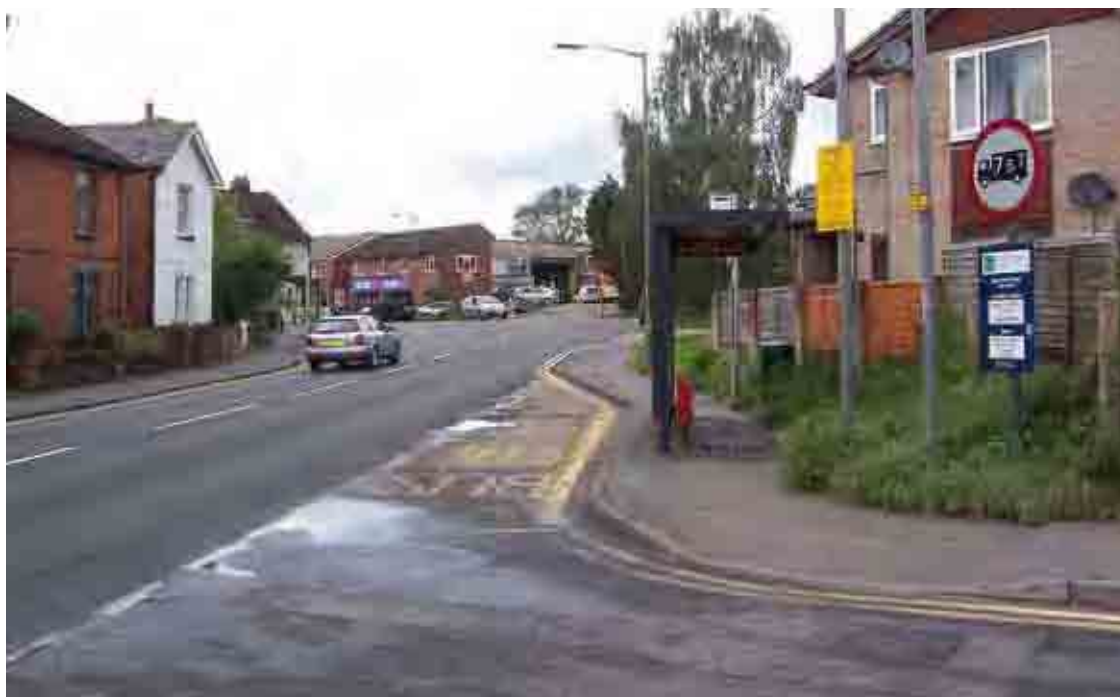
Figure 6.17 The bus lay-by facilitates the free movement of other vehicles, but it is inconvenient for pedestrians.
